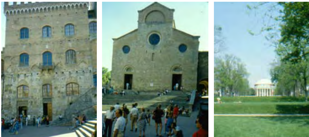
Figures 14, 15 and 16. Horizontal and vertical themes in architecture; starting from the left, the Town Hall and church in San Gimignano, and on the right the University campus in Charlottesville.
